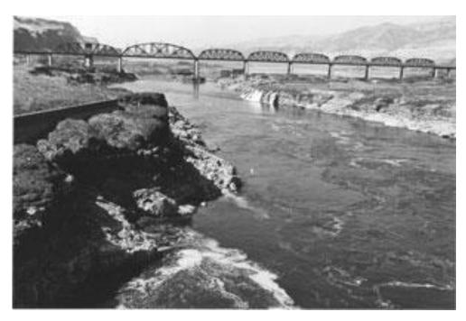
The Army Corps of Engineers built the Dalles-Celilo canal which provided passage around Celilo Falls and the Long Narrows until The Dalles Dam replaced it in 1957. *Courtesy of the Army Corps of Engineers.*
